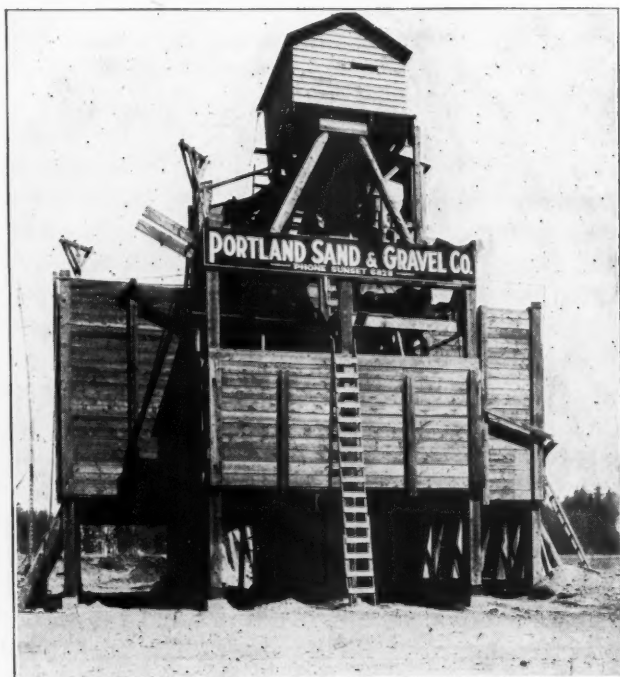
The Storage and Screening Plant Right on a Section Line Highway
